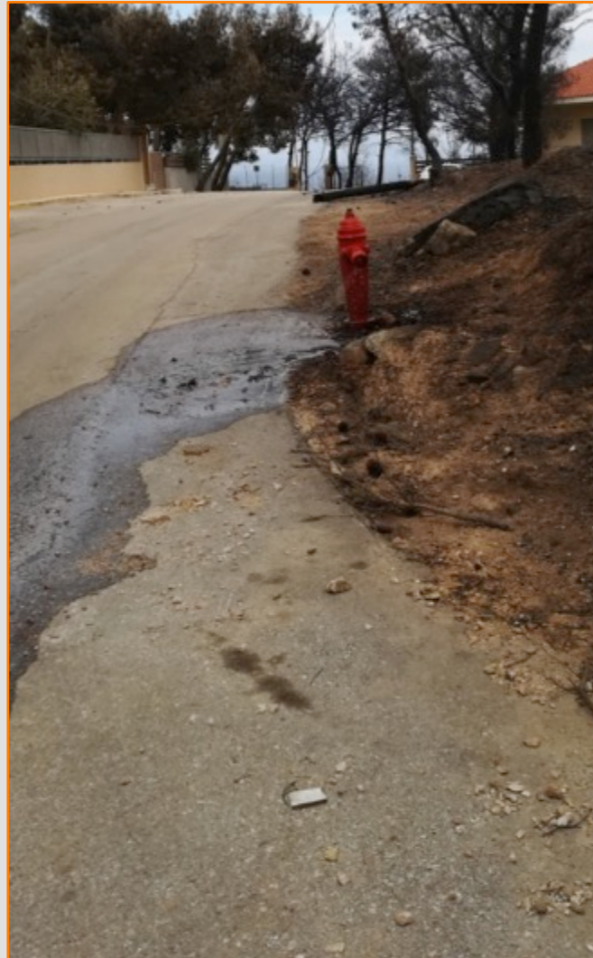
Damage on the water network of the fire-affected area
